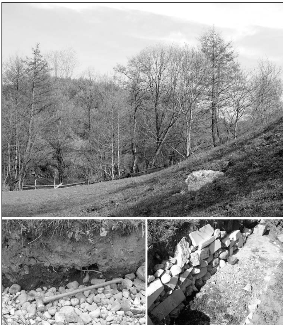
Fig. 3. Ex situ experimental plot in the vicinity of Dobrinishte in the foothill of Pirin Mts. – drainage layer and stonework with marble peaces.
